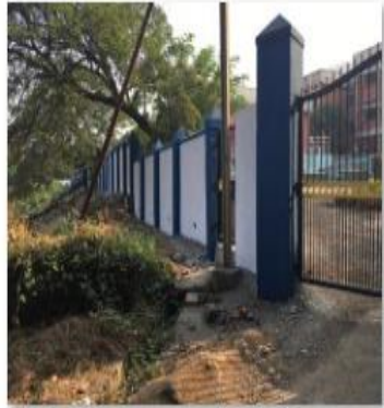
Boundary Wall and Gate
